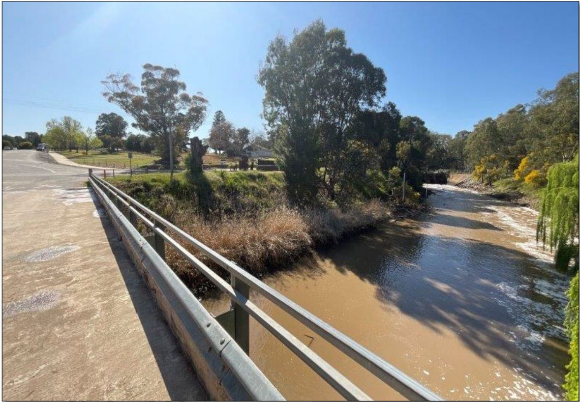
Plate 9: Bundidgerry Creek and irrigation channel
