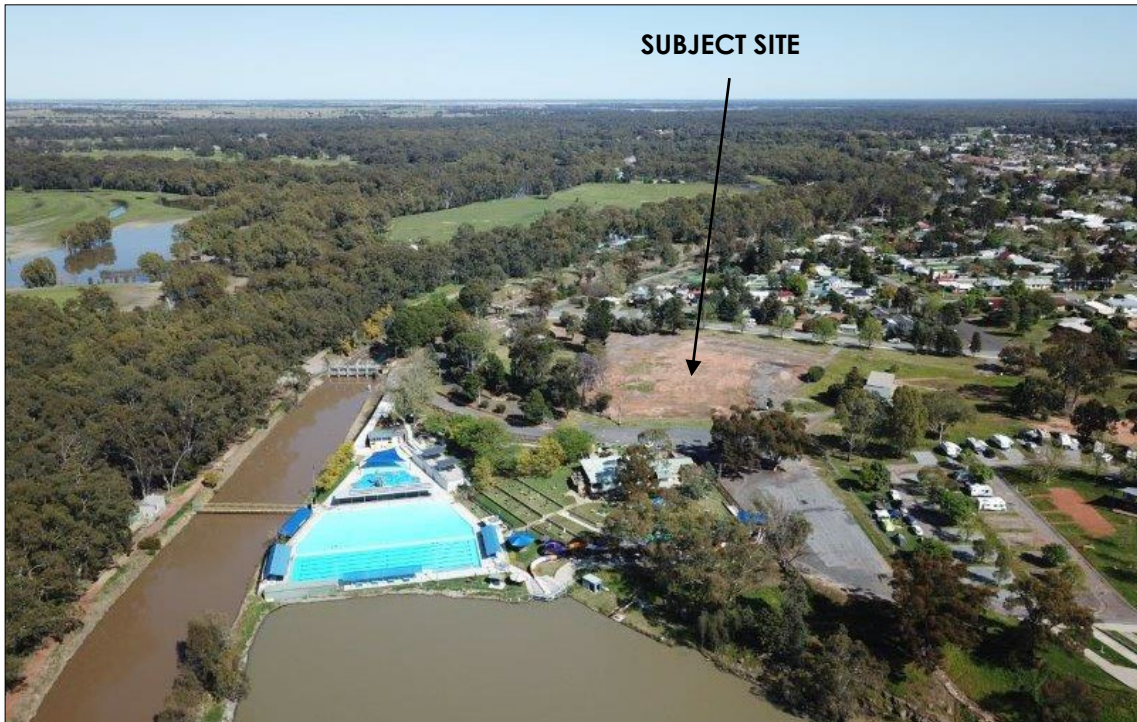
Plate 5: Looking west over public swimming pool
