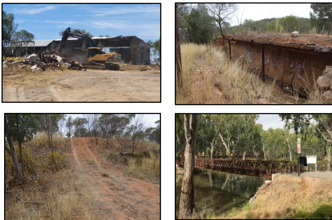
Figure 6: Areas of Reserve 81121 (including during Holcim site demolition)
