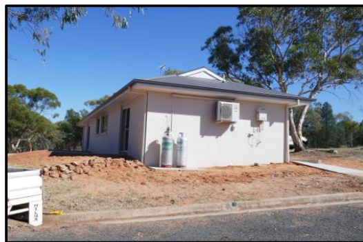
Newly refurbished 2 x 2 bedroom motel units.
