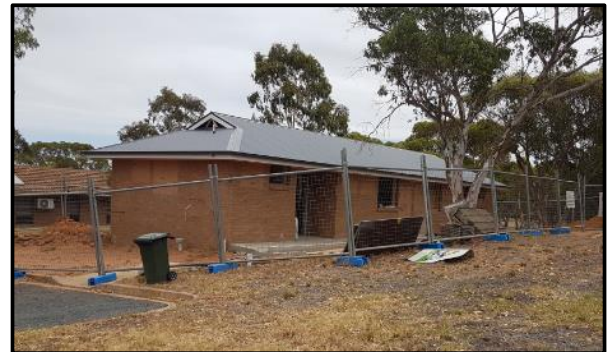
New residential building in progress
