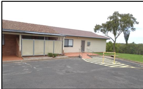
New disabled access motel unit (insurance funded)
